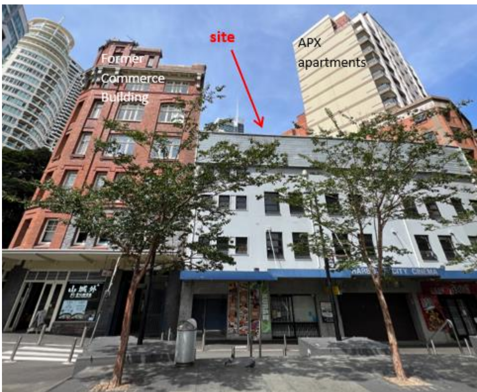
Figure 7: View to the rear of the site (behind the Harbour City Cinema) from Day Street facing east
