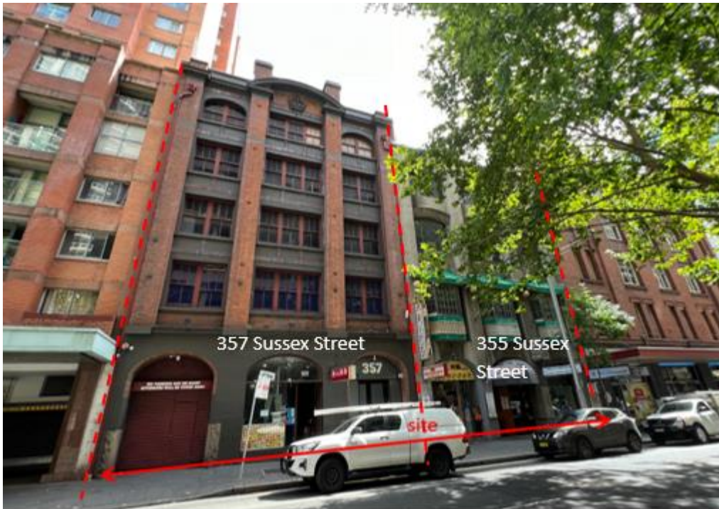
Figure 2: Site viewed from Sussex Street facing west
