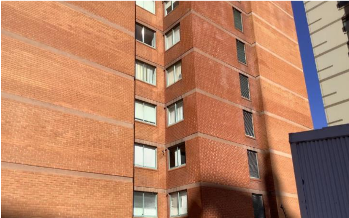
Figure 57: Existing northern lightwell (bedroom windows) of the Regal Apartments viewed from the subject site facing south
