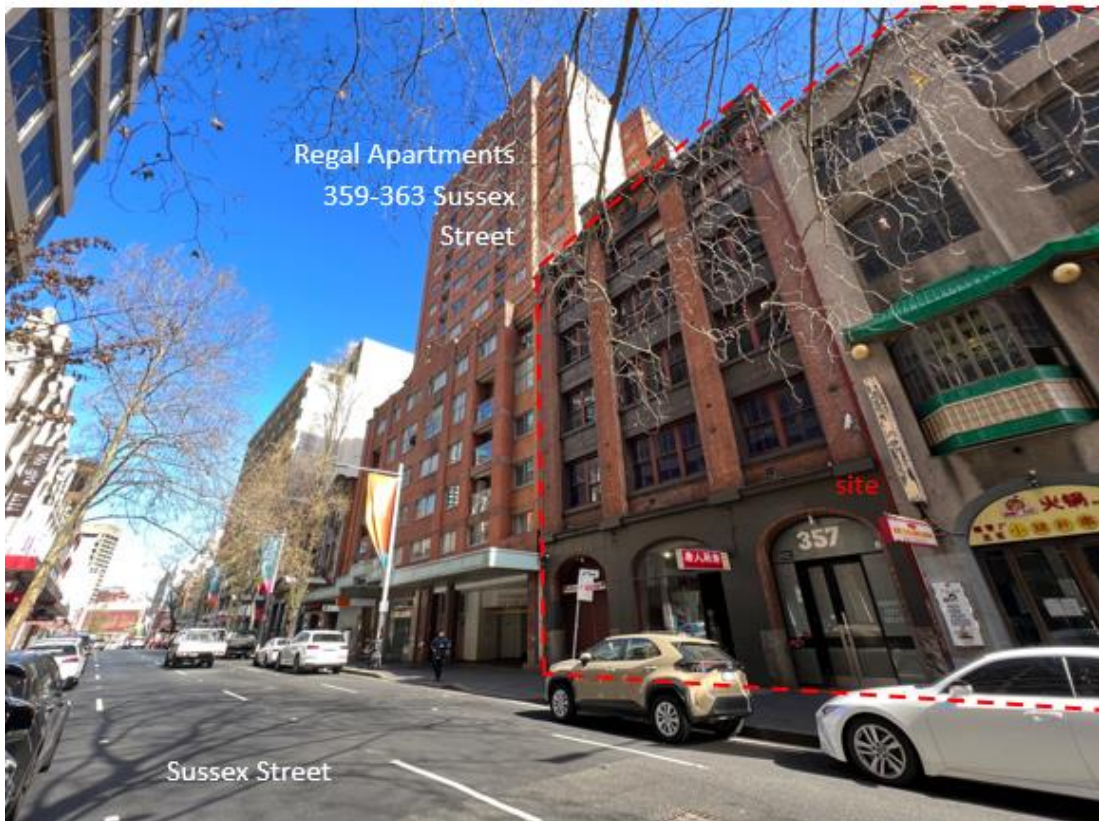
Figure 10: View of the site and southern adjoining developments on Sussex Street facing south
