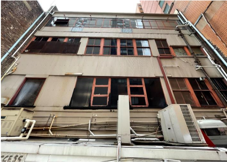
Figure 4: Existing rear elevation of 357 Sussex Street facing east
