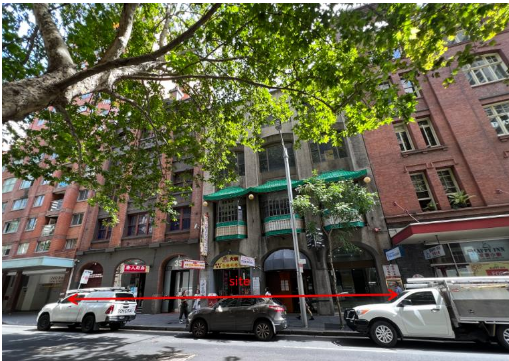
Figure 3: Site viewed from Sussex Street facing west
